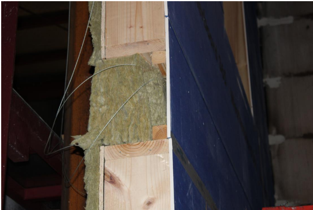
Photo No. 4 Internal thermocouples was mounted in the gap and wired out through the side.
