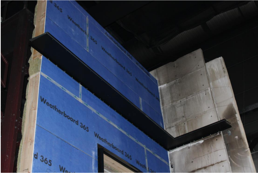
Photo No. 5 The pre painted flame deflectors was mounted above the gaps spanning further out than the wall.
