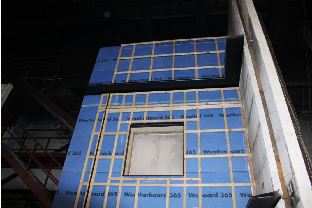
Photo No. 7 Vertical and horizontal formworks was mounted
