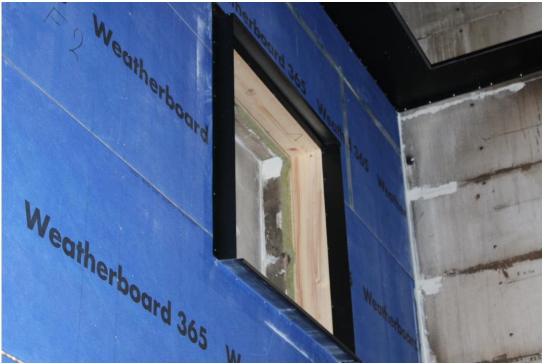
Photo No. 6 Pre painted steel mounted around the window.
